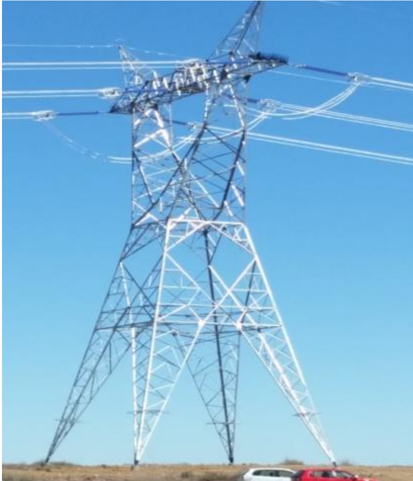
517E SELF SUPPORTING STRAIN TOWER
