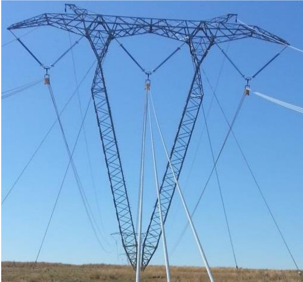
520B GUYED VEE SUSPENSION TOWER
