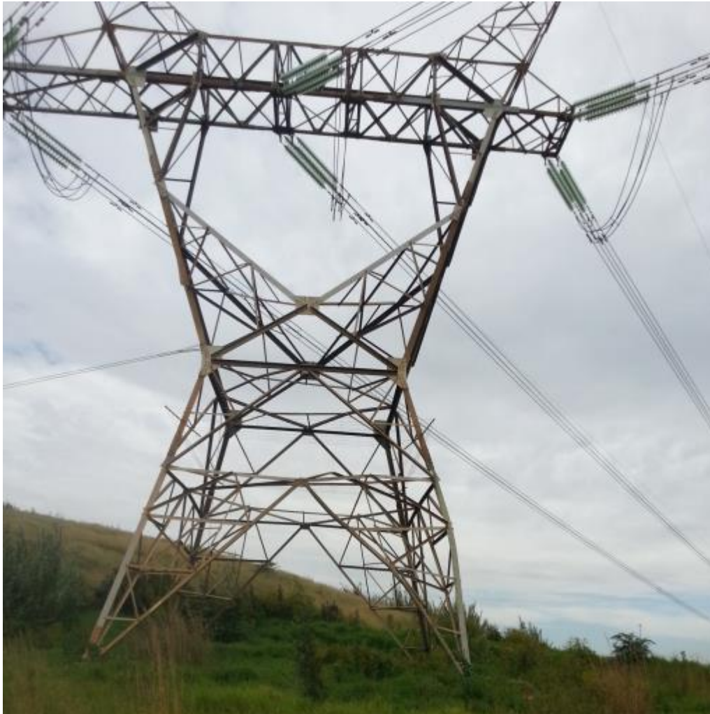
275KV SELF SUPPORTING STRAIN TOWER-433E-DESIGNED FOR QUAD ZEBRA
